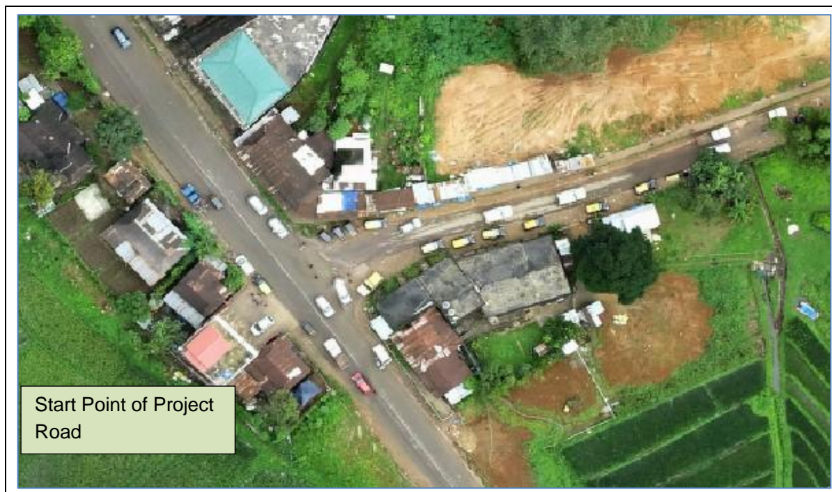
Figure 2: Start Point of Project Road at Junctions of the NH-6/ AH road
